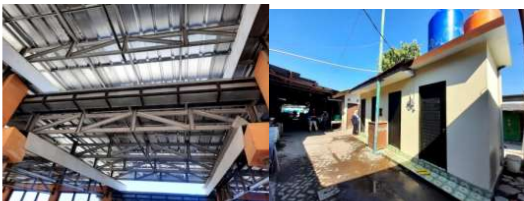
Rehabilitasi Pasar Bantul
